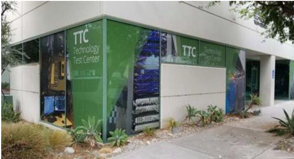
SCE Technology Test Center (TTC)
